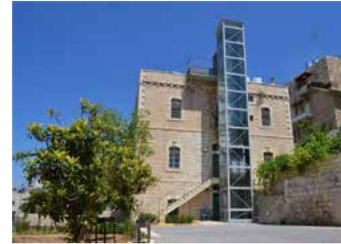
Eastern elevation of the Marcos Nassar building, showing the steel and glass external elevator.
