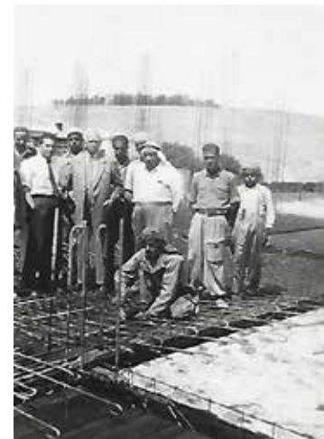
Nadia's father with coat and tie inspecting the iron reinforcement. He often sent Nadia to check it, but what does a little girl know!!! The house no longer exists. It may have been unfinished and belonged to Anton Batato in Upper Baqa'a.
